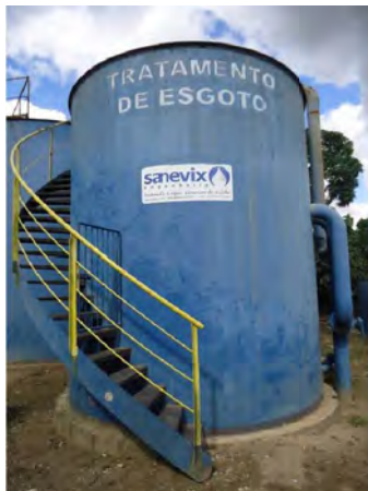
(c) Reator aeróbio
